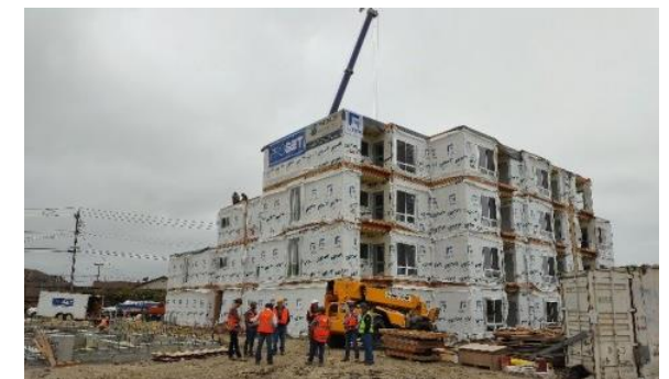
Parkside Manor Phase I Construction
