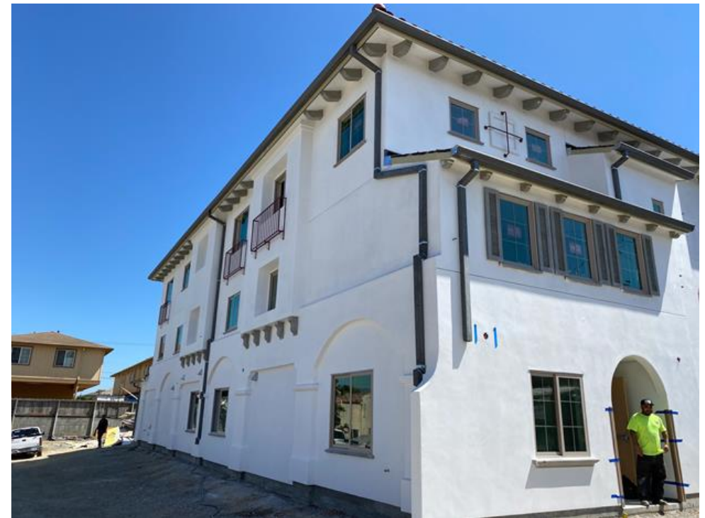
Sun Rose Apartments Construction
