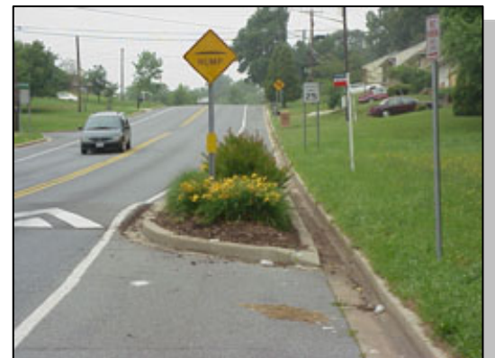
Example: Retrofit design with unimpeded drainage.
