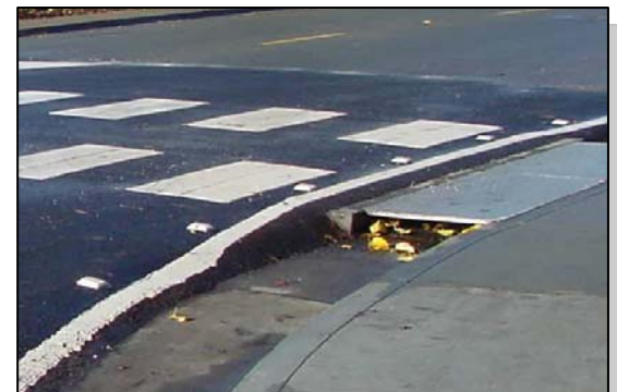
Example: Unimpeded drainage.
