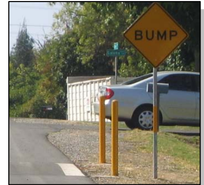
Example: Bollards and advisory sign encourage drivers to travel over speed hump.
