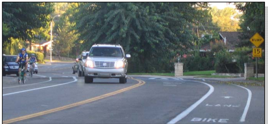
Example: Speed lump extends to the edge of pavement across bike lane.
