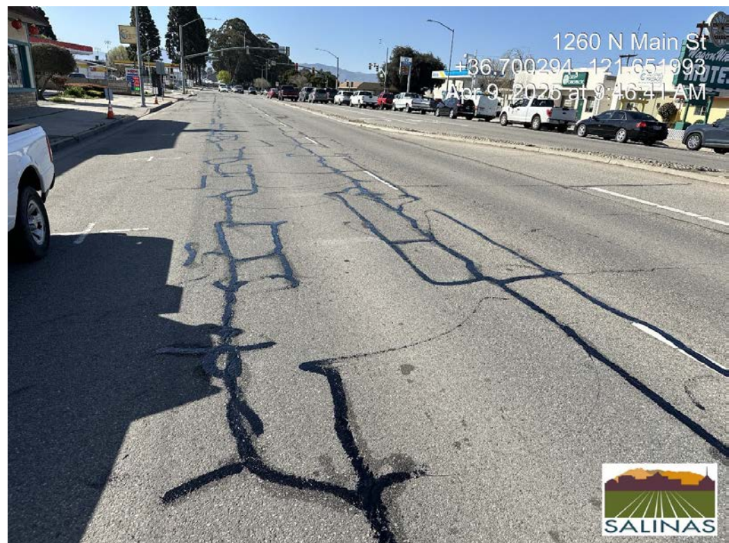
Crack Treatment – N. Main St.
