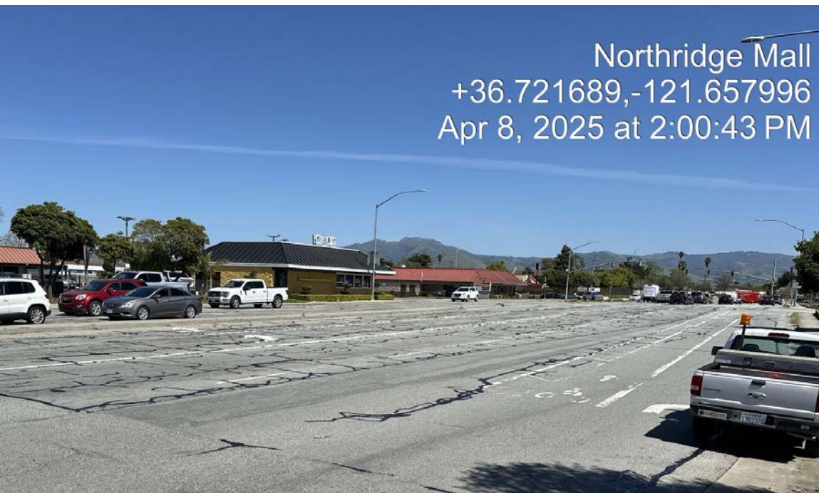
Crack Treatment Boronda Rd
