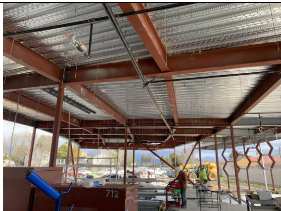
Completed fire sprinklers level 1
