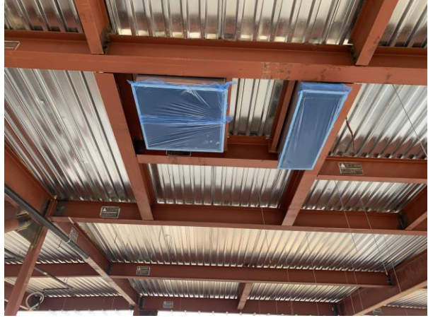
Duct drops through roof deck from rooftop A/C units
