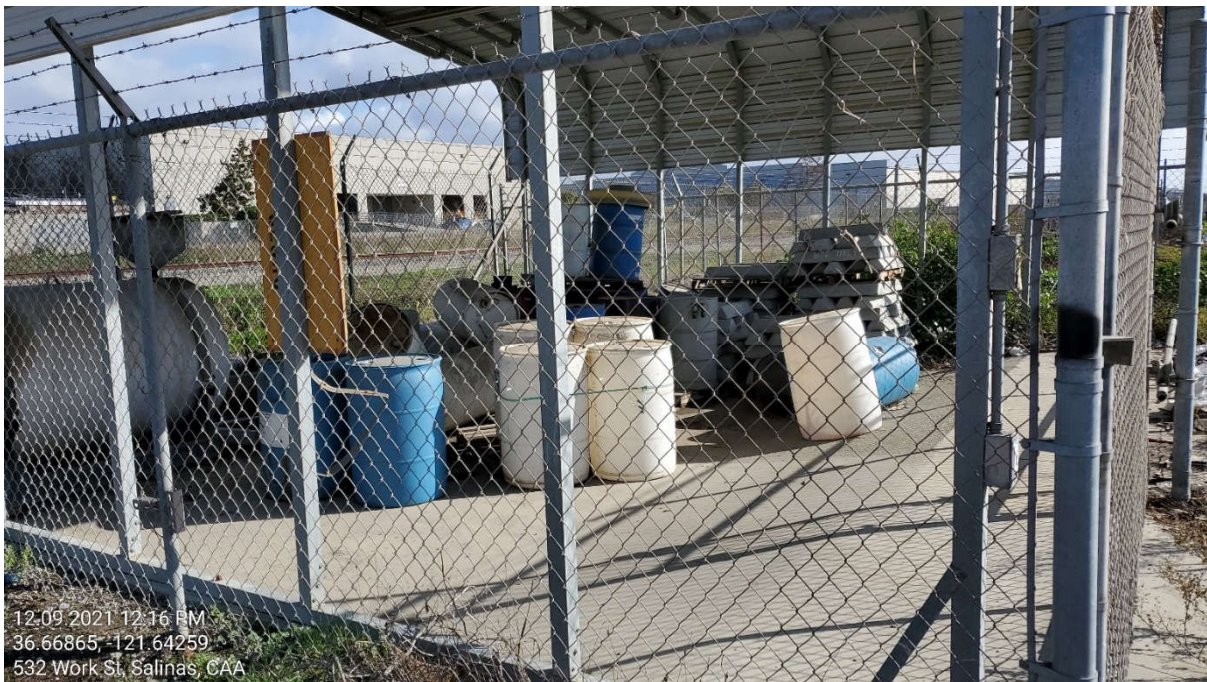
Photograph 4. View of a hazardous materials storage area in the southeastern corner of the project site (near the 348 Abbott Street building) with an aboveground storage tank (AST), drums, and buckets.
