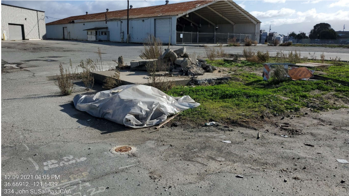
Photograph 5. View of the area of the former diesel underground storage tank (UST) in the central-eastern portion of the project site. A groundwater monitoring well is visible.
