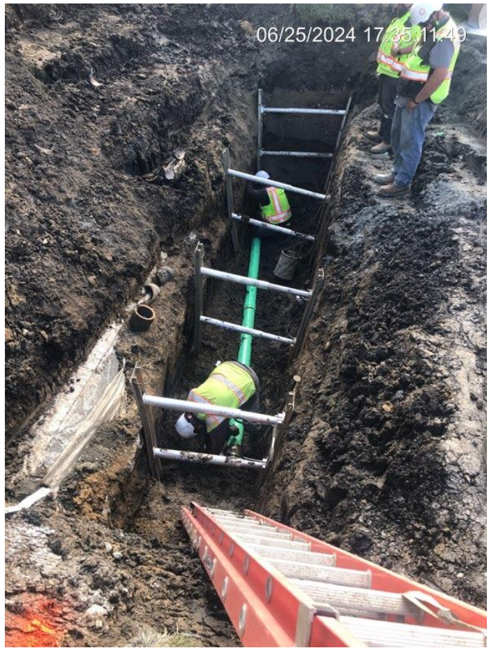
Image 7. Sewer Main Repair
