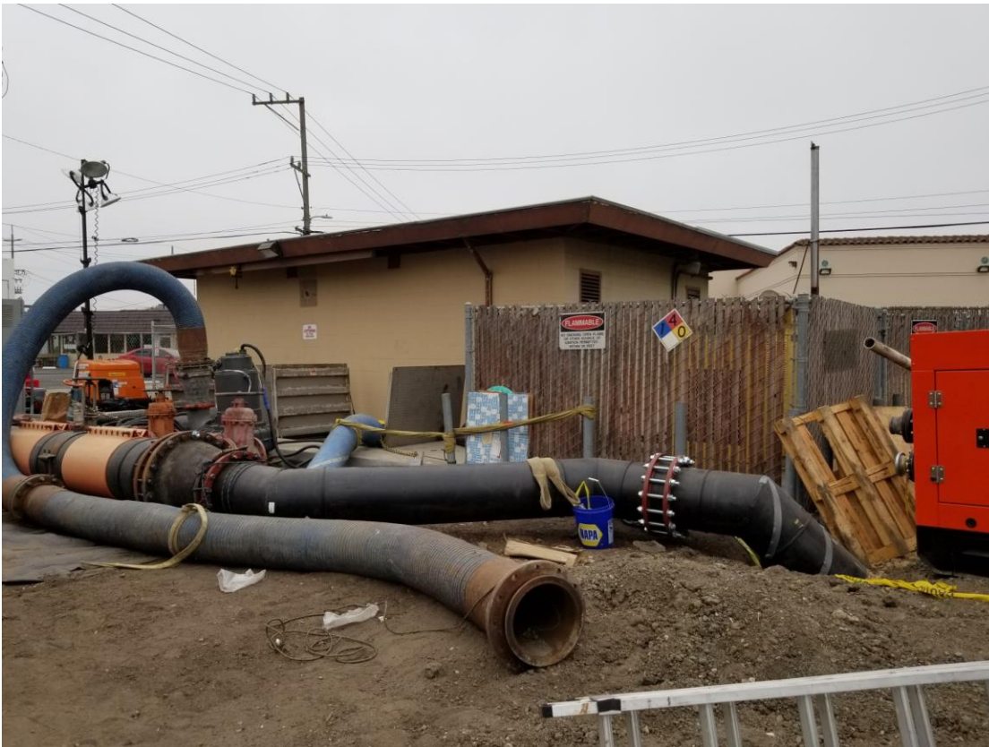
Image 8. Sewer Bypass for Sewer Main Replacement
