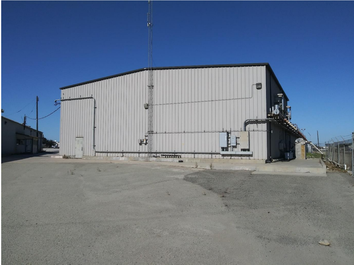
Figure 8 View north of the south elevation of Building 3
