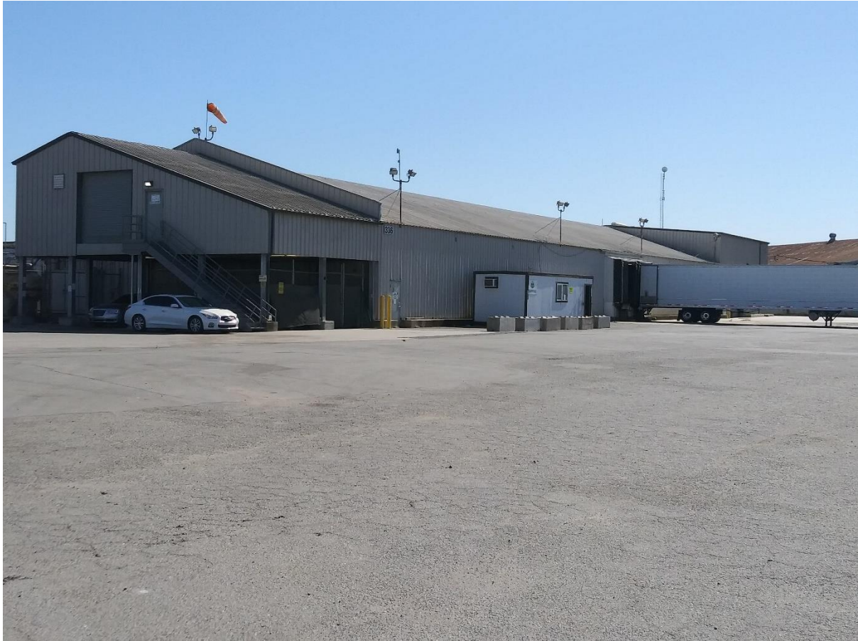
Figure 9 View southeast of the north and west elevations of Building 3
