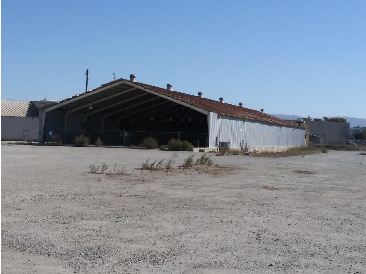
Figure 6 View southeast of the west and south elevations of Building 2
