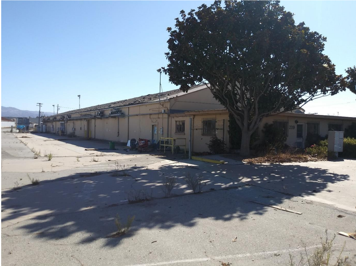
Figure 4 View southeast of the west and north elevations of Building 1
