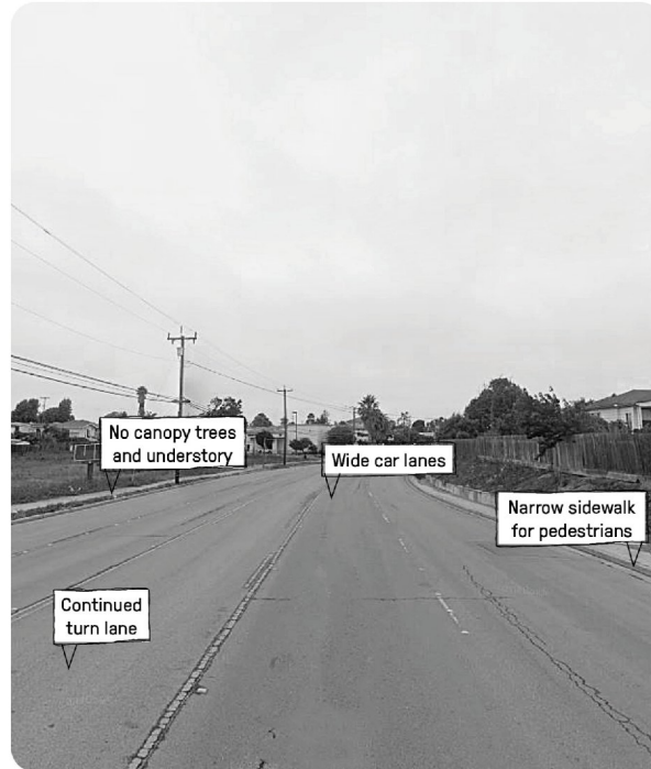
Typical road condition at AVP opportunity zone in Sanborn Rd
