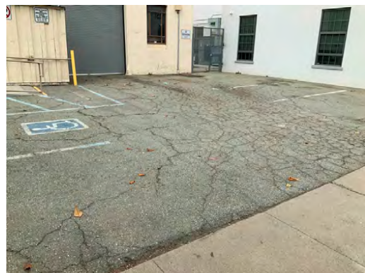
East parking area deteriorated asphalt
