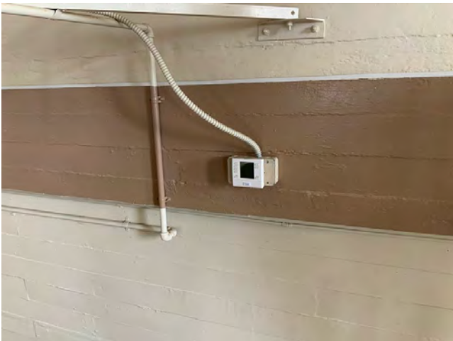
95. Space heater thermostat
