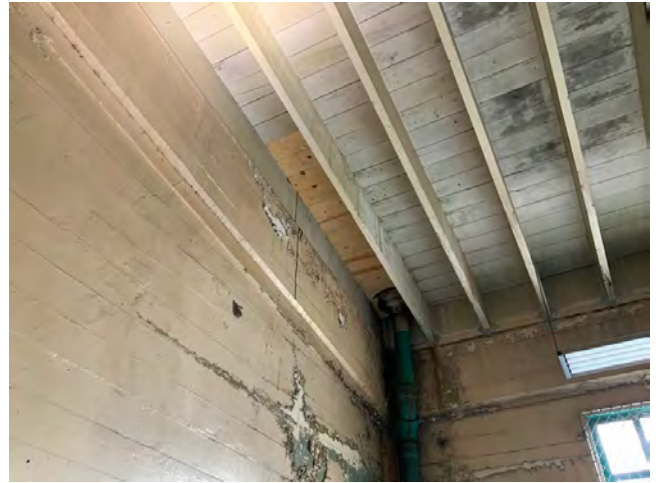
30. Repaired roof decking
