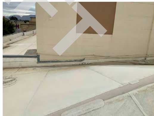
Unattached sections of the north roof
