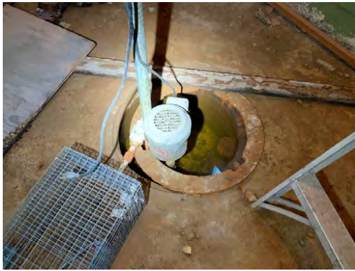
Basement sump pump
