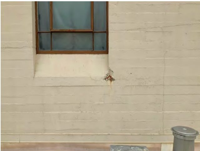
39. Exterior wall exposed rebar
