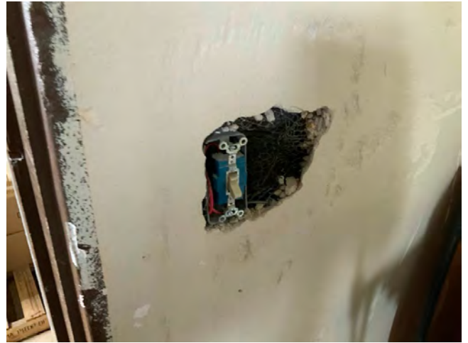
102. Exposed electrical wiring
