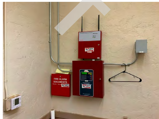
Fire alarm panel and communicator
