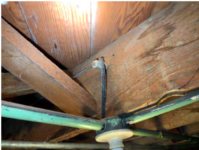
103. Knob and tube wiring
