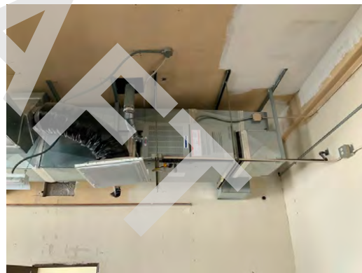
Ceiling hung gas-fired furnace
