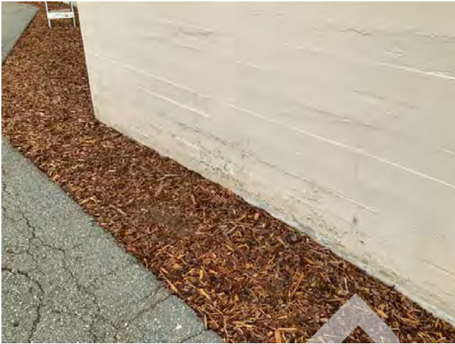
37. Peeling exterior paint
