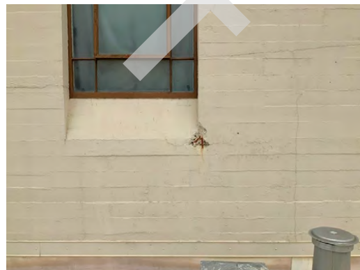
Exterior wall exposed rebar
