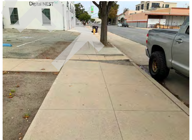
132. Public sidewalk displacement
