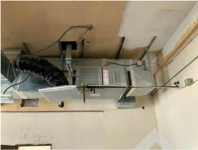
97. Ceiling hung gas-fired furnace
