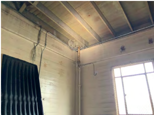
167. Roof drainage
