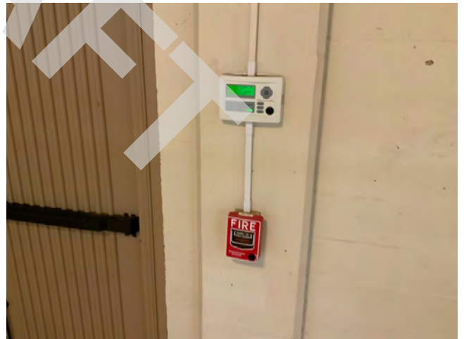
112. Fire alarm annunciator panel and pull station
