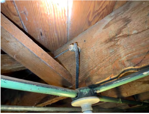
Knob and tube wiring
