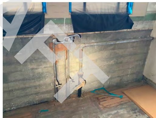
Possible galvanized piping
