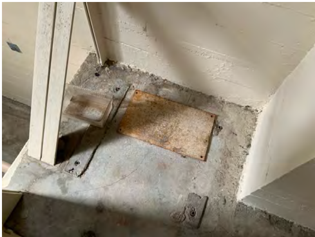
67. Concrete hole covered with plywood
