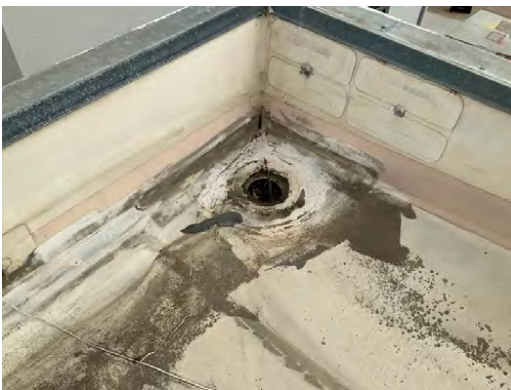
Missing roof drain dome
