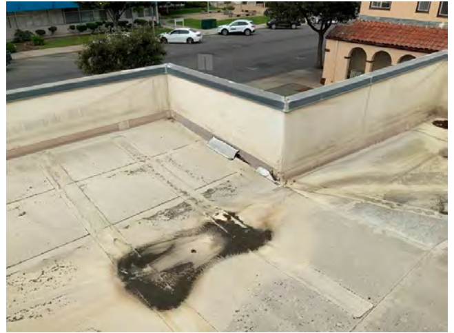
54. Roof patchwork and low spots
