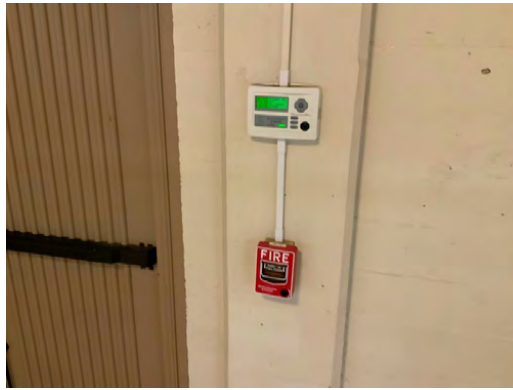
Fire alarm annunciator panel and pull station
