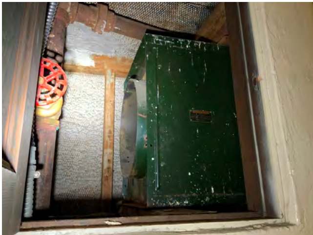
183. Decommissioned hydronic fan coil unit
