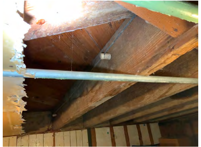
162. Knob and tube wiring
