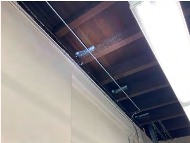
151. Lower roof support brackets
