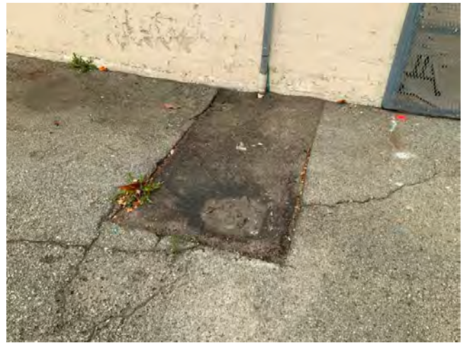
138. Asphalt repair patch
