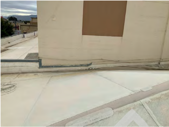
57. Unattached sections of the north roof
