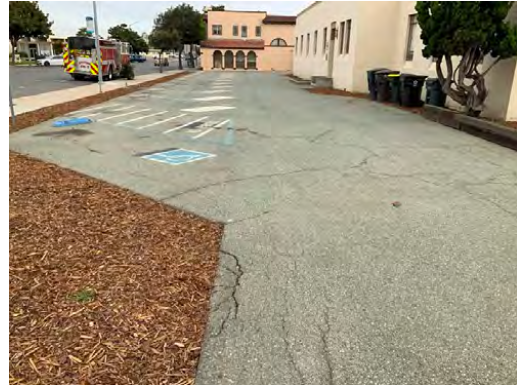
West parking lot cracking
