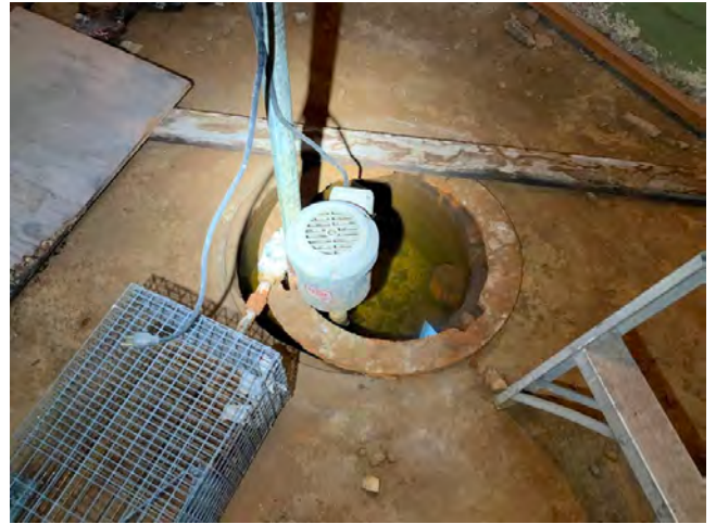
90. Basement sump pump
