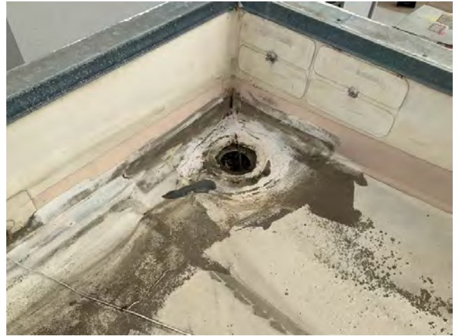
50. Missing roof drain dome
