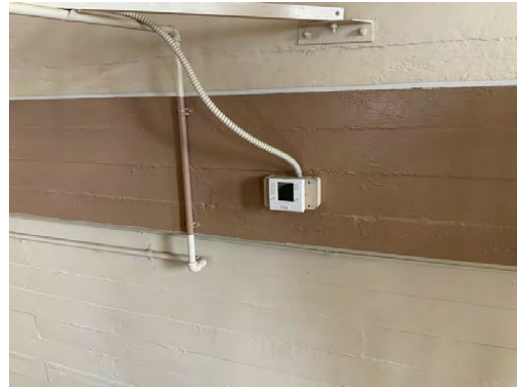
Space heater thermostat
