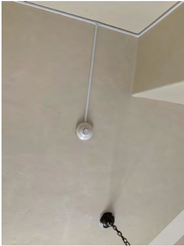
157. Ceiling mounted smoke alarm
