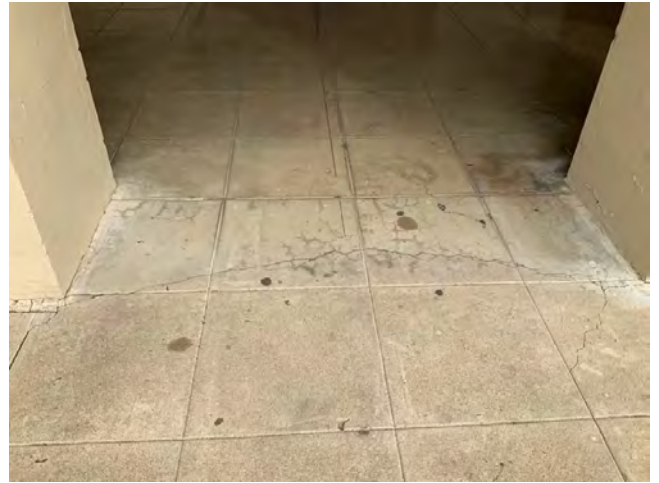
142. Cracking concrete flatwork
