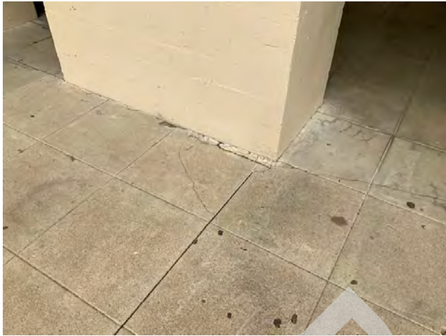
141. Cracking concrete flatwork
