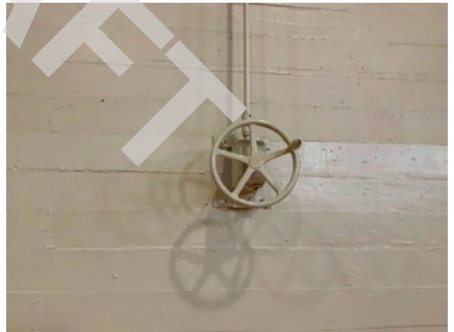
100. Controls for operable windows
