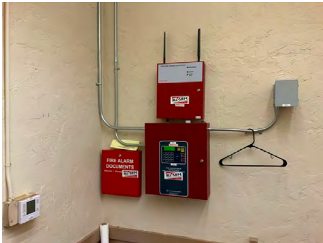
111. Fire alarm panel and communicator
