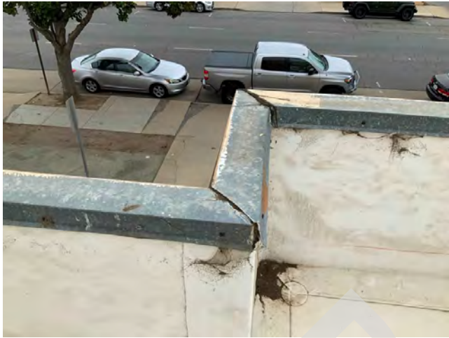
45. Coping missing sealant
