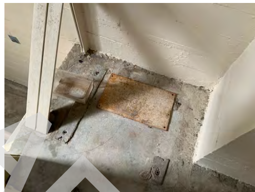
Concrete hole covered with plywood
