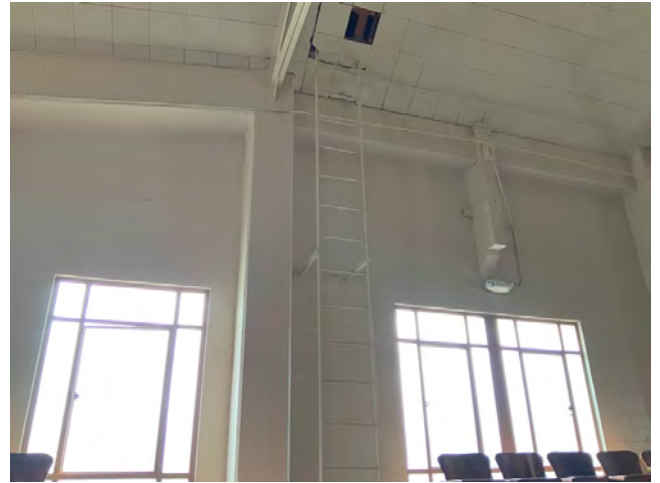
146. Upper roof access ladder
