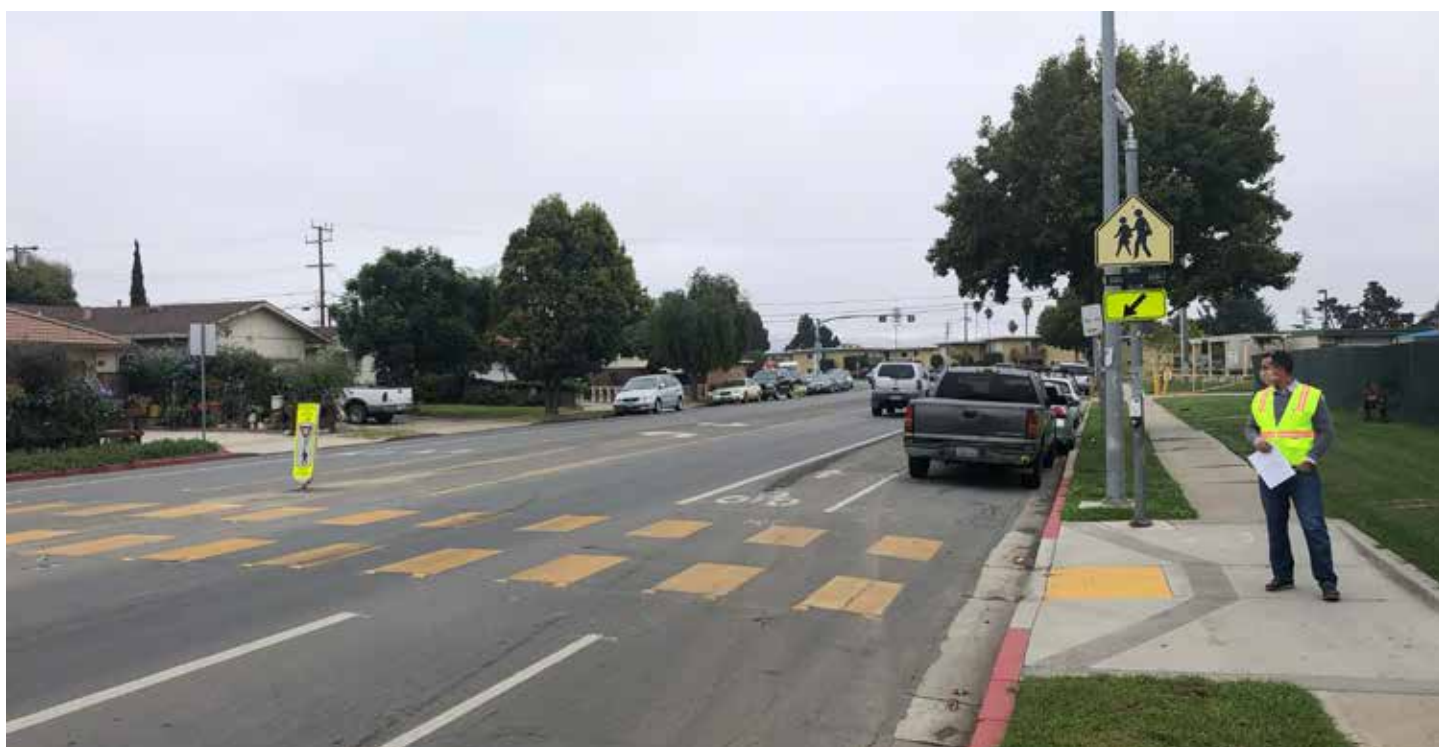
A road diet, bike lanes, and rectangular rapid flashing beacons were installed on John St
