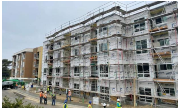
Parkside Manor Phase I - Construction
