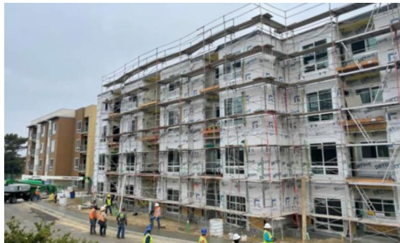
Parkside Manor Phase I - Construction
