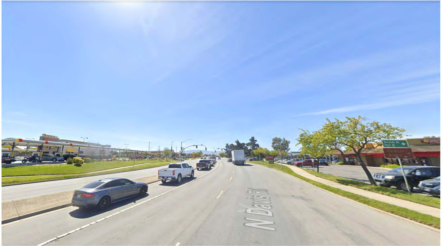
Figure 4-2 Mountain Ranges to the South North Davis Road, looking south (cross street: Prader Street). Source: Google Earth 2021
