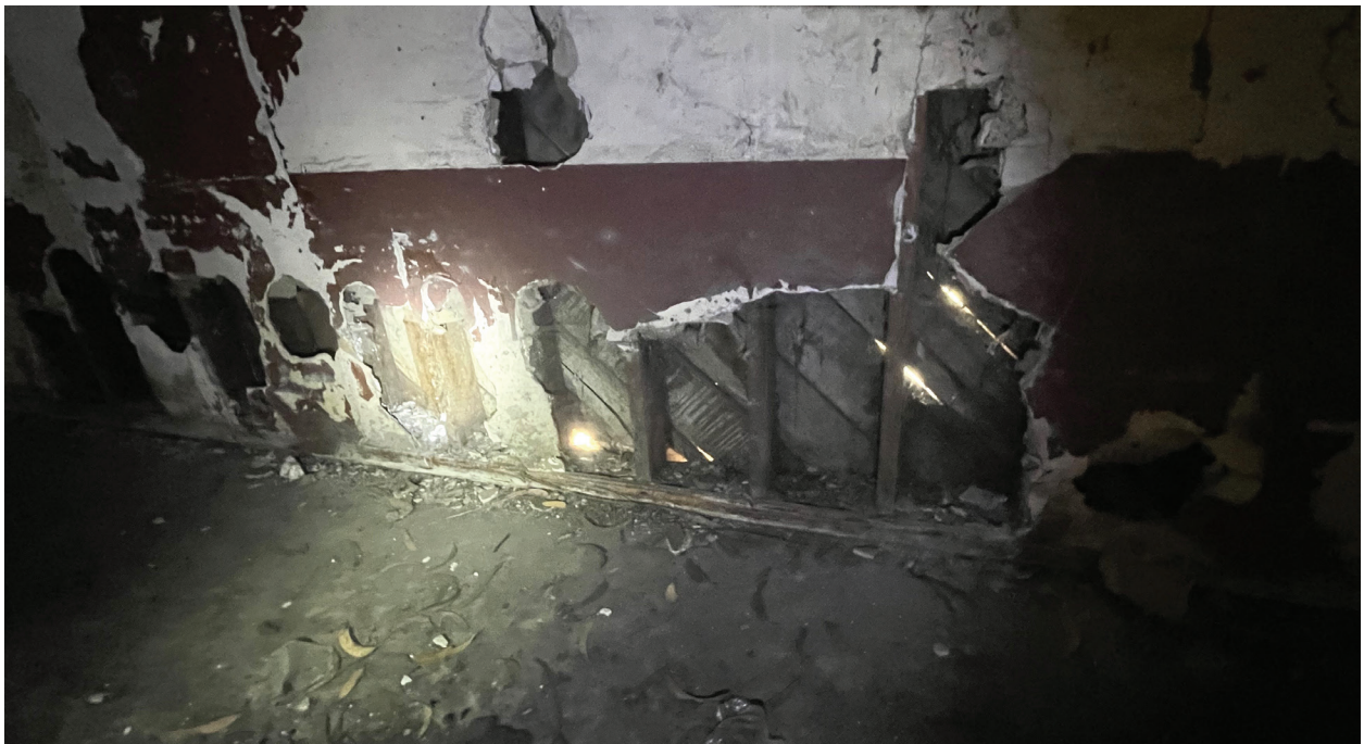
Figure 5.23 Large sections of gypsum board have been damaged along the south elevation, Groundwork Preservation, LLC, 2024.
