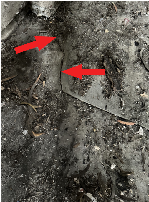
Figure 4.2 Photo of minor damage to the concrete floor slab near the north wall, Howard Carter Associates, Inc, 2024.
