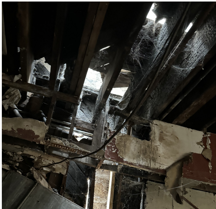
Figure 4.3 Photo of wood floor joist connection to wood wall framing at the south wall, Howard Carter Associates, Inc, 2024.
