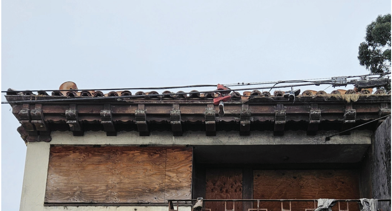
Figure 5.7 The barrel clay tile roof on the east facade is in poor condition. The decorative metal gutter is missing a large portion and has many plants growing from it, TEF Design, 2024.
