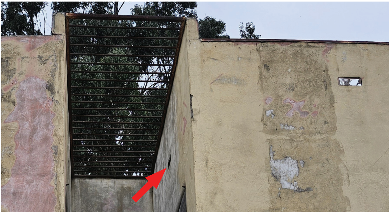
Figure 5.4 The metal through wall scupper seen here serves as drainage to the deck of the lightwell, typical of both lightwells, TEF Design, 2024.
