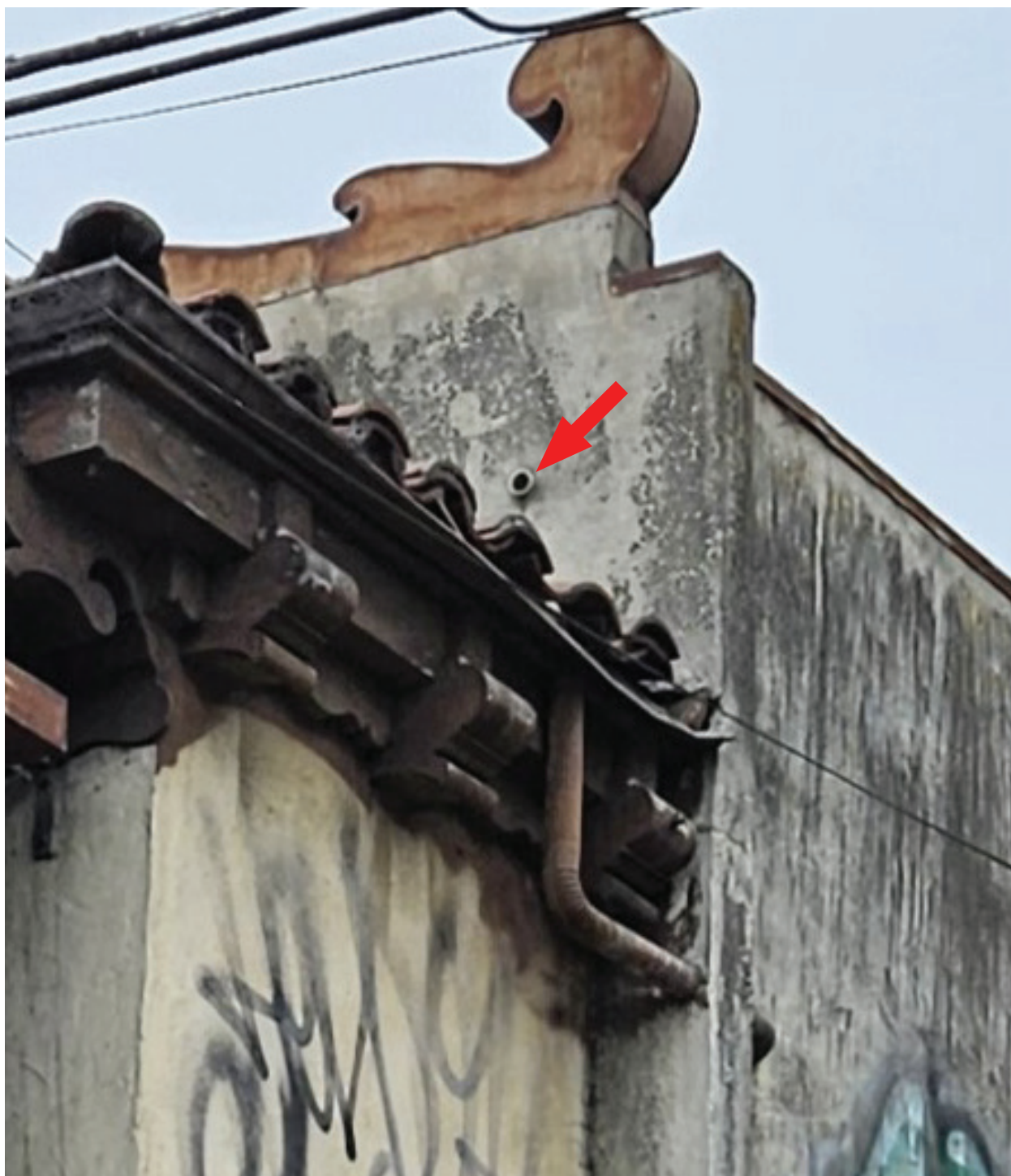
Figure 5.6 A small, round through wall metal scupper presumably drains water from the main roof to the hipped clay tile roof at the east facade, TEF Design, 2024.
