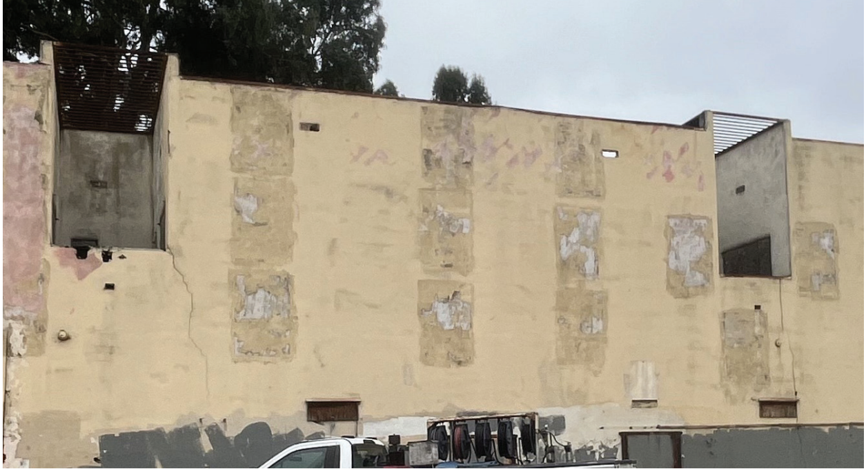
Figure 5.3 Large rectangular openings through the parapet wall of the south facade and lightwell walls may provide drainage for the flat roof of the building, TEF Design, 2024.
