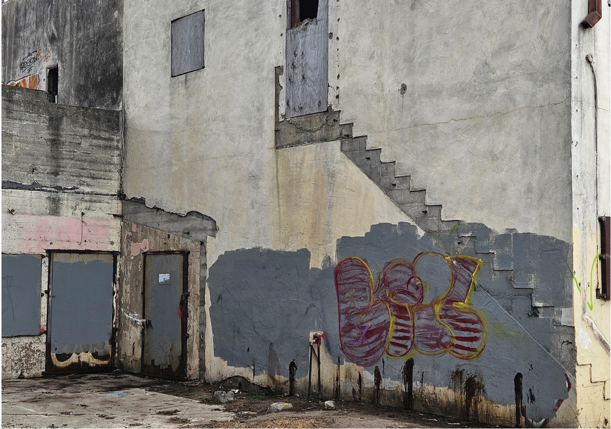
Figure 5.13 Portions of the stucco at the west end of the north facade are missing where previously attached architectural components have been removed, TEF Design, 2024.
