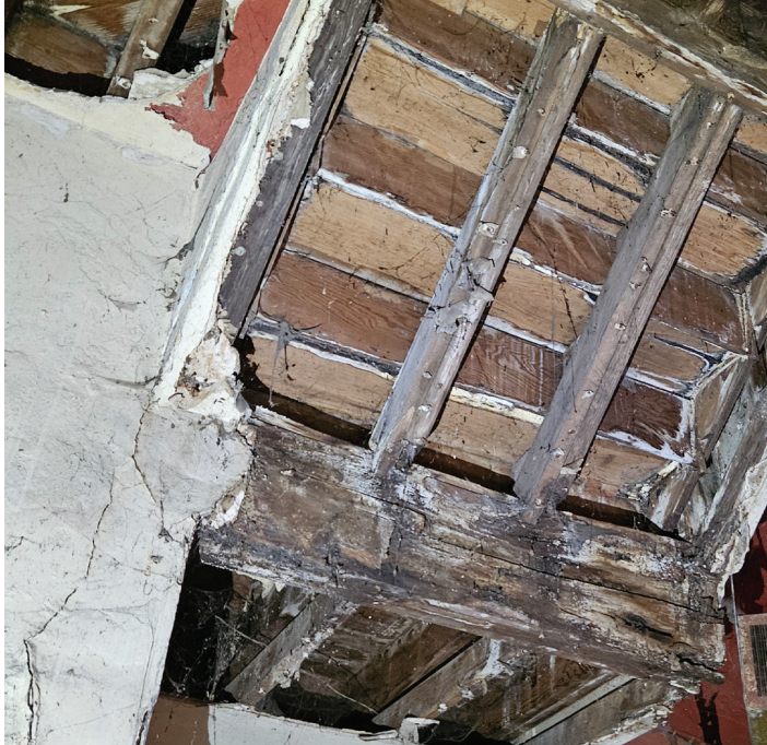
Figure 5.24 The landing at the stair to the second floor is unsupported at the outer corner. The framing is deteriorated from water intrusion, TEF Design, 2024.
