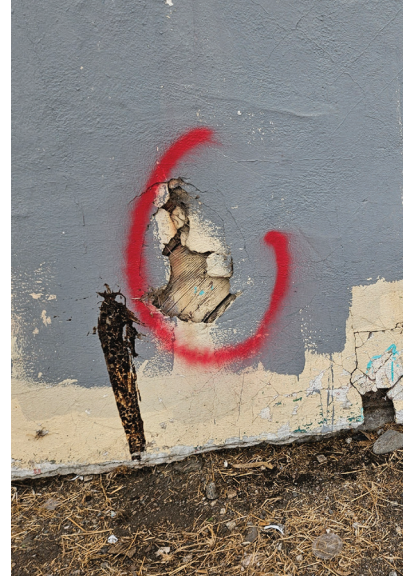
Figure 5.16 Detail view of stucco deterioration at the south facade, TEF Design, 2024.
