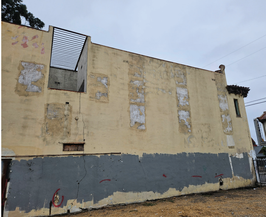
Figure 5.19 This view of the east end of the south facade reveals many additional areas of failing stucco, TEF Design, 2024.
