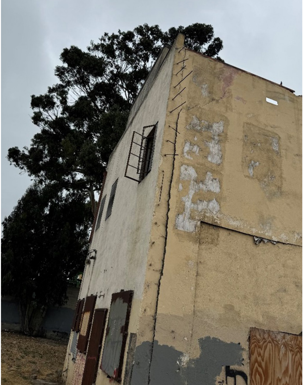
Figure 4.6 Photo of full height crack in stucco at southwest junction of concrete wall and wood framed wall, Howard Carter Associates, Inc, 2024.
