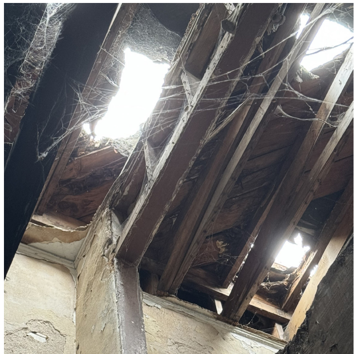
Figure 4.5 Photo of roof wood truss framing and failing roofing above, Howard Carter Associates, Inc, 2024.
