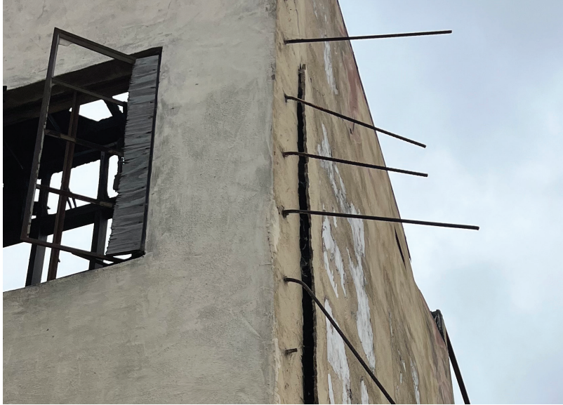
Figure 5.15 The stucco has pulled away from the wall and reinforcement protrudes at the south west corner, TEF Design, 2024.
