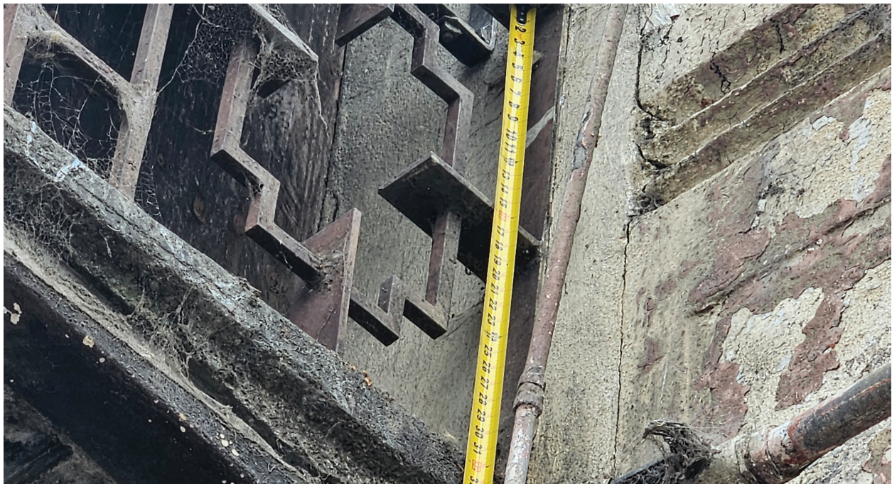
Figure 5.12 The decorative metal railing at the balcony is only 32 inches high, TEF Design, 2024.
