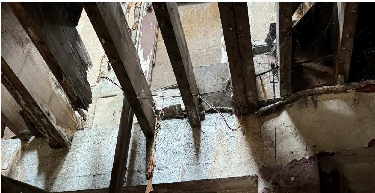
Figure 4.4 Photo of wood floor joist connection to concrete ledger at the north wall, Howard Carter Associates, Inc, 2024.
