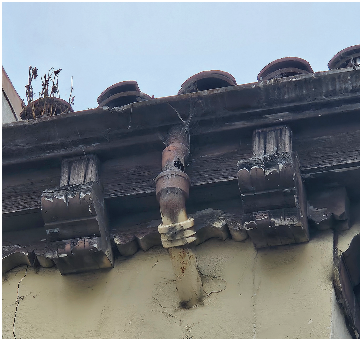
Figure 5.8 On the south side of the clay tile hipped roof, tiles are broken and shifted. The downspout at this facade is rusted with a large hole, TEF Design, 2024.
