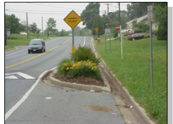
Example: Retrofit design with unimpeded drainage.
