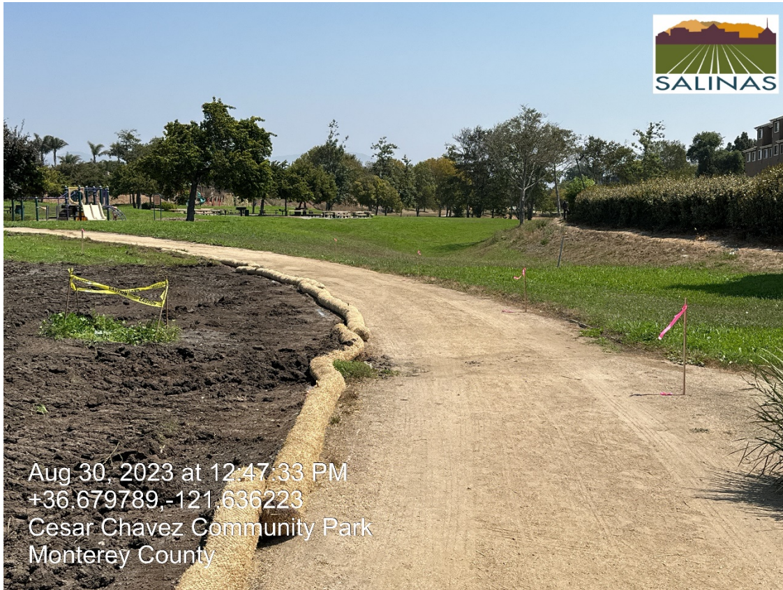
During Construction – Bioretention Area
