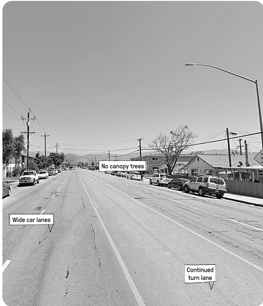
Typology 1. Typical existing road condition at residential land use in Williams Rd
