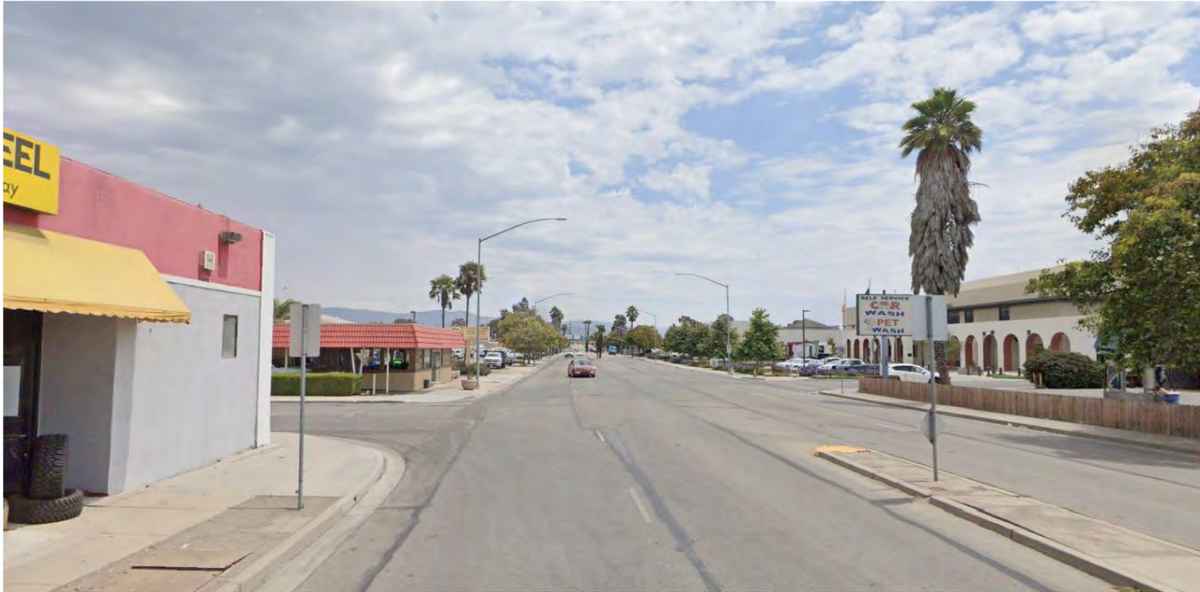
Figure 4-2 Mountain Ranges to the East East Alisal Street, looking east (cross street: Prader Street). Source: Google Earth 2022
