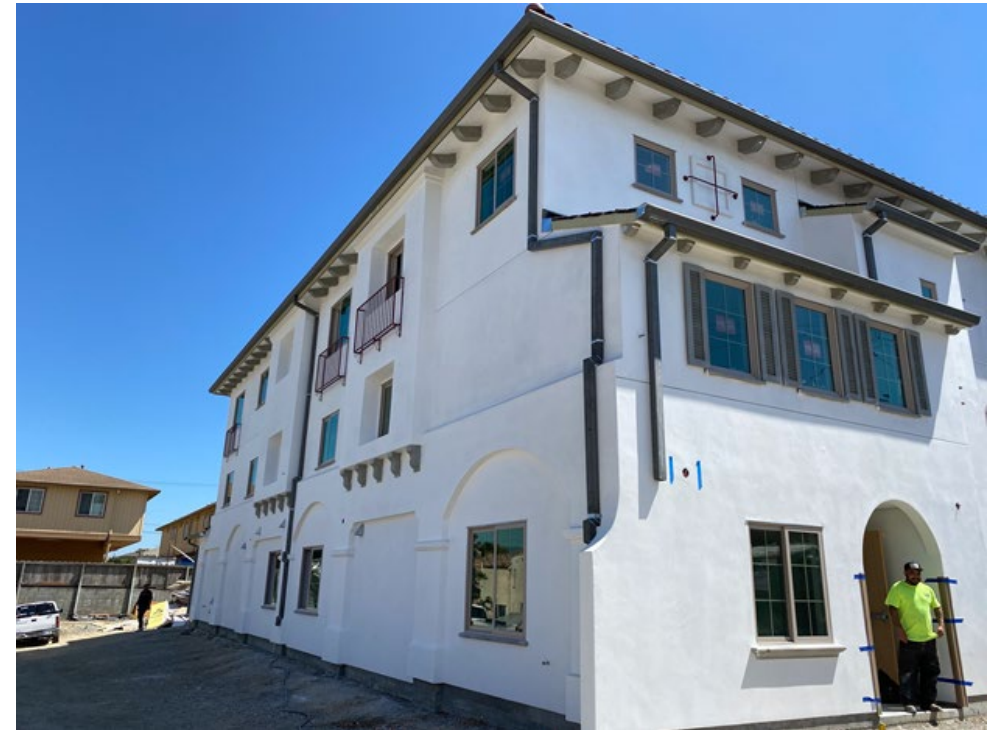
Sun Rose Apartments Construction
