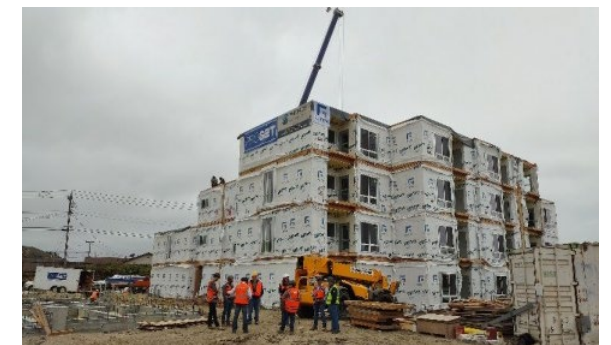
Parkside Manor Phase I Construction
