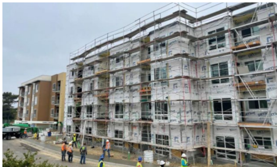
Parkside Manor Phase I Construction
