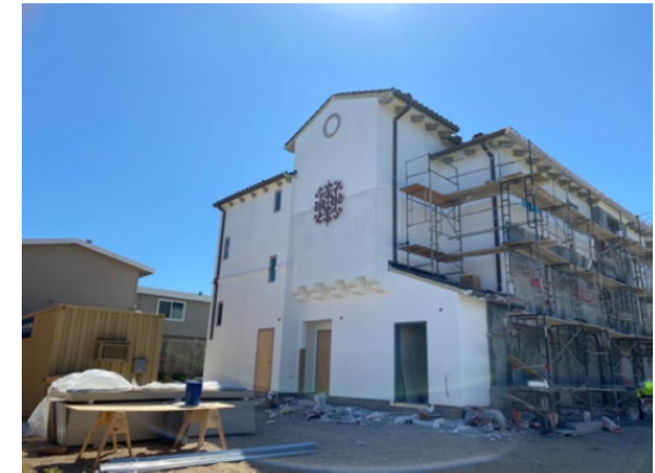
Sun Rose Apartments Construction
