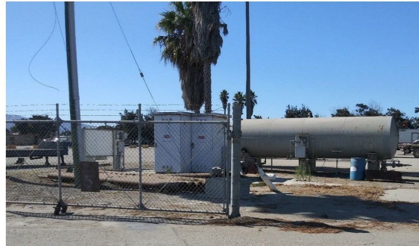
Northern portion of site facing west towards existing storage tank
