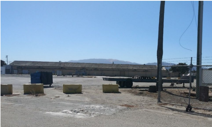
Northwestern portion of site facing south towards Building 1
