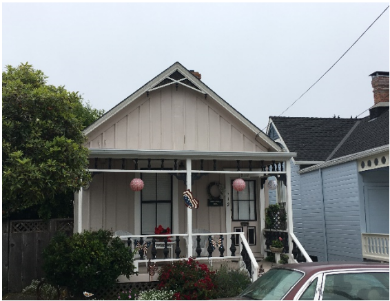
Figure 15: A narrow tent cottage with board and batten cladding and limited Victorian-era decorative detailing at 112 18 th Street. Source: Page & Turnbull, August 2, 2018.
