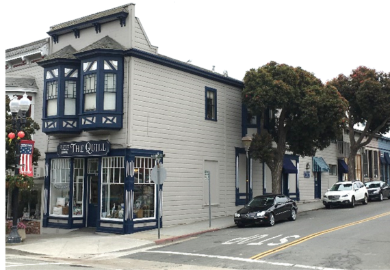
Figure 7: A row of commercial buildings on Lighthouse exhibit the typical Western Non-Contributor Front commercial style. Although originally one-story buildings, these buildings were enlarged as Pacific Grove grew and retain integrity to the period of significance. Source: Page & Turnbull, August 3, 2018.
