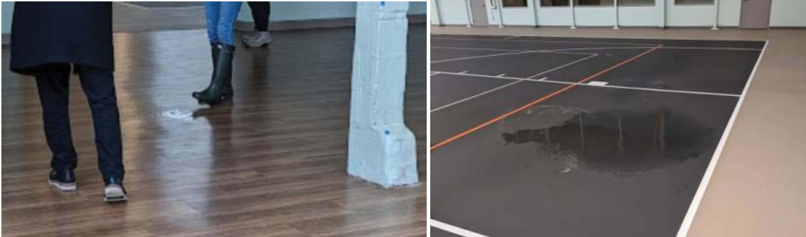
Water observed at SE corner of gym
