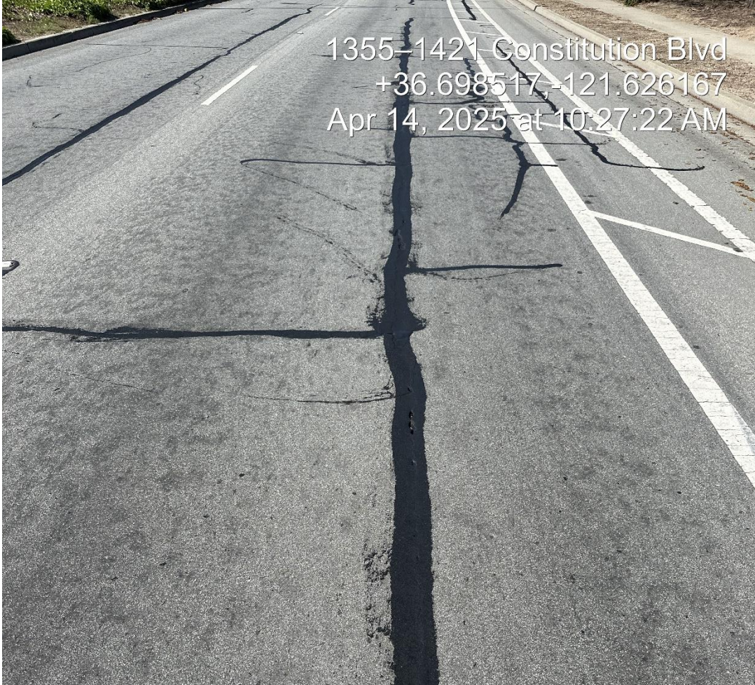
Crack Treatment – Constitution BLVD
