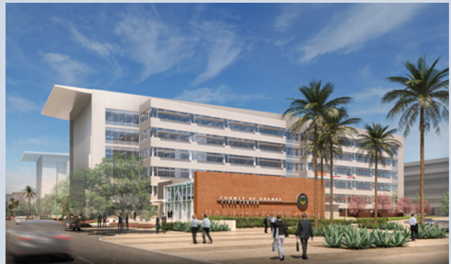
County of Orange, Building 16
