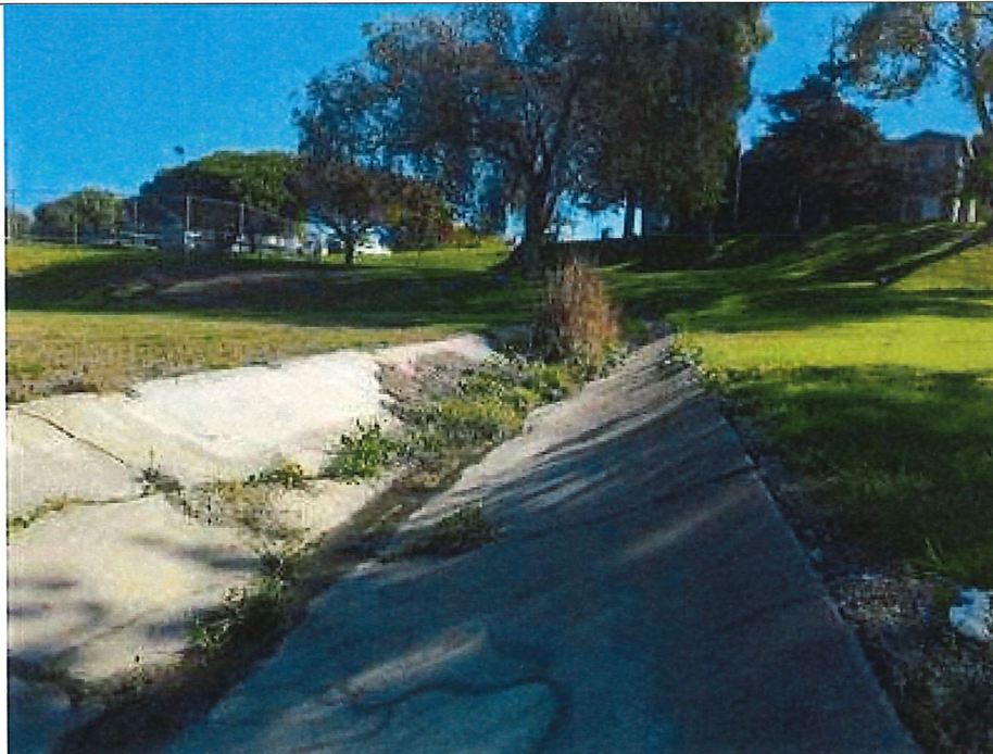
Photograph 4: (36.686362, -121.656581) Cement-lined V-ditch that drains uplands west towards AR-01. View facing east.
