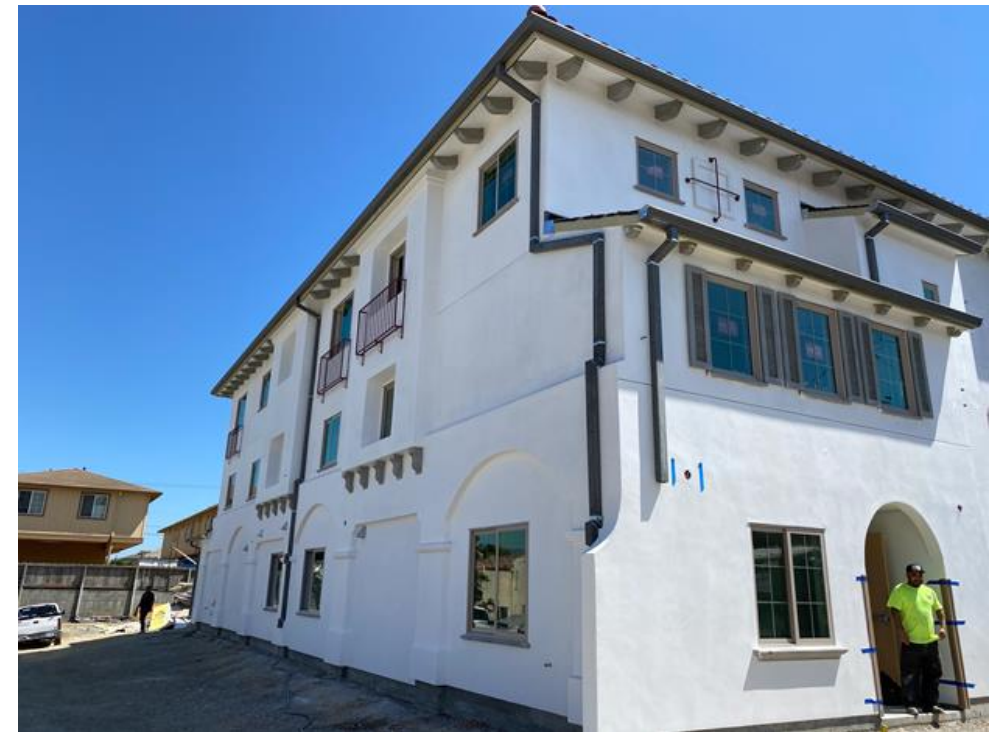
Sun Rose Apartments Construction
