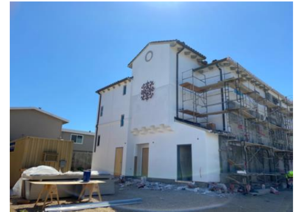
Sun Rose Apartments Construction
