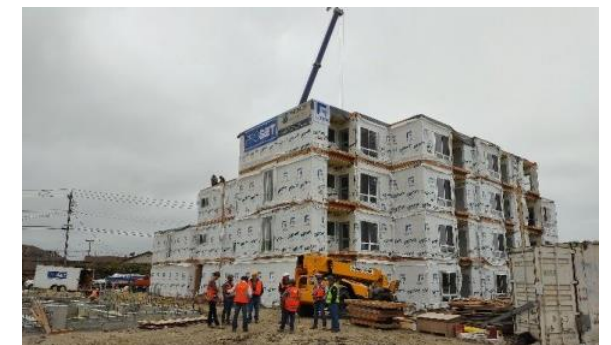
Parkside Manor Phase I Construction
