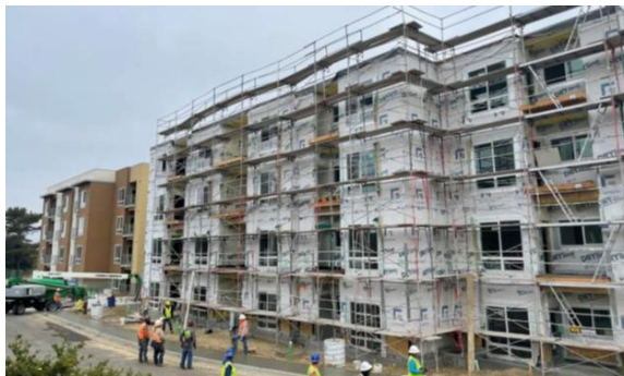
Parkside Manor Phase I Construction
