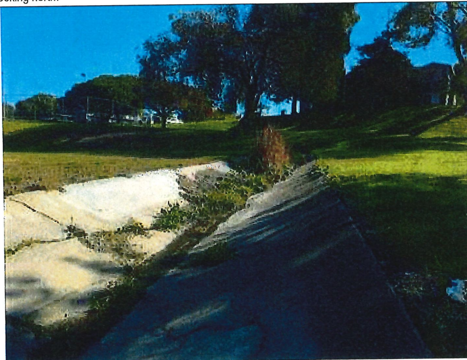
Photograph 4: (36.686362, -121.656581) Cement-lined V-ditch that drains uplands west towards AR-01. View facing east.
