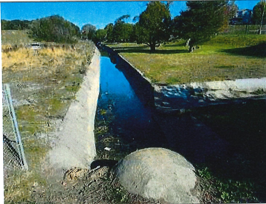
Photograph 1: (36.686279, -121.656684) AR-01 flowing just east of the project SITE, with a cement-lined v-ditch on the right-hand side of the photo. View facing north.
