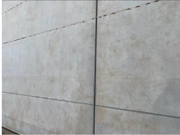
Most wall panel accent reveals are properly aligned
