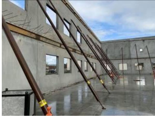
Two story walls temporarily braced
