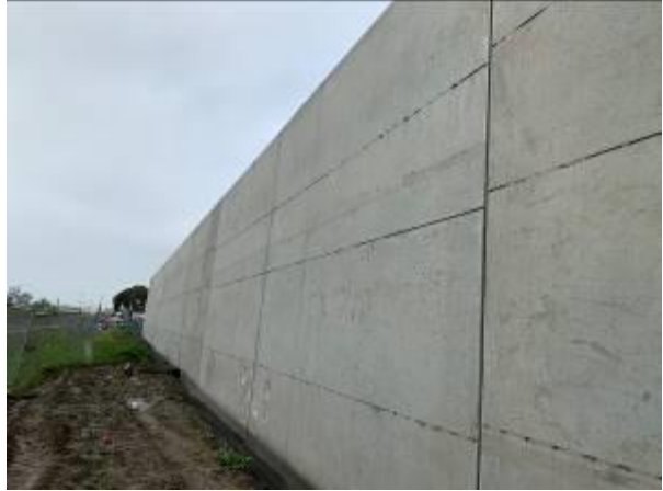
Two panels have misaligned reveals, will need repair
