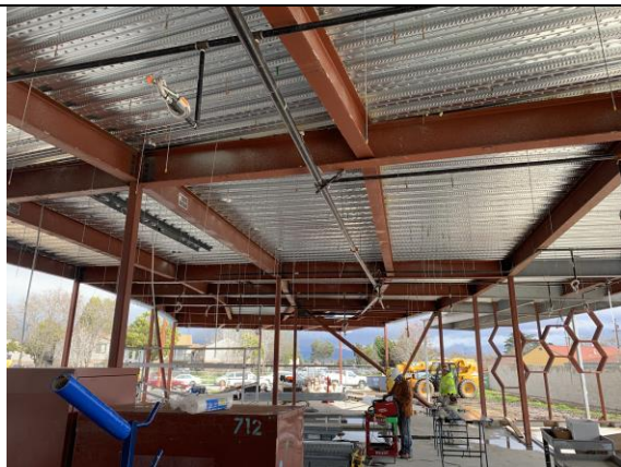
Completed fire sprinklers level 1
