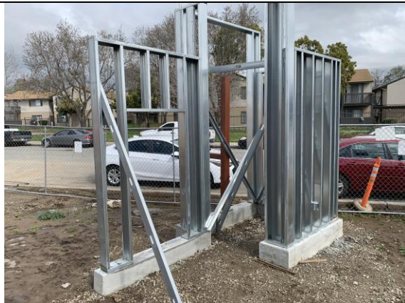
Exterior wall mock up framed
