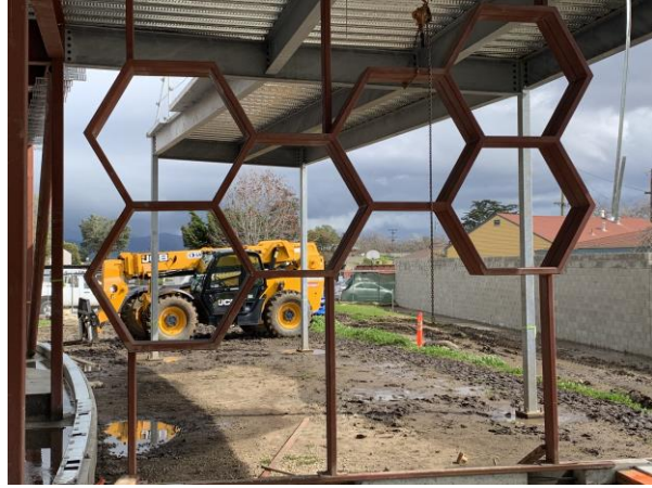
Art wall support installed
