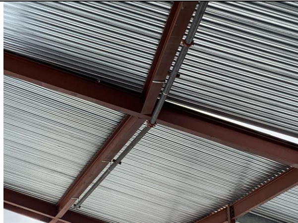
Floor 2 sprinkler main started
