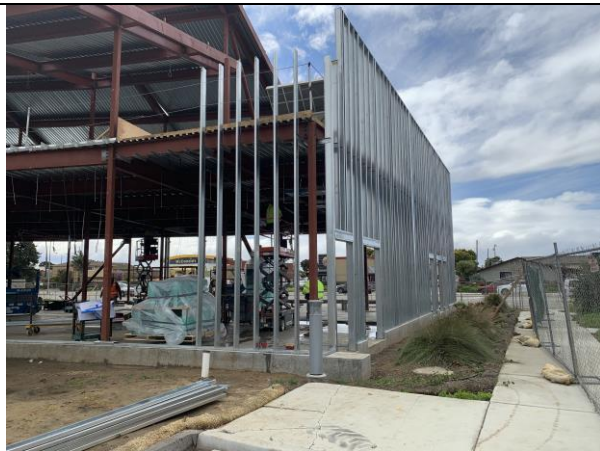
North wall framing in place
