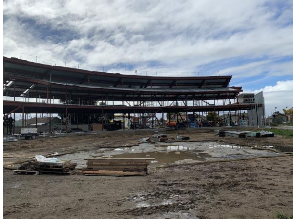
Steel decking spread over 98% of roof framing
