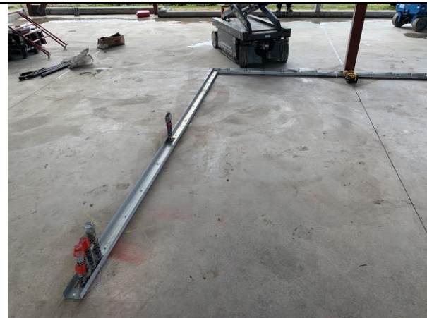
First floor wall framing lower track
