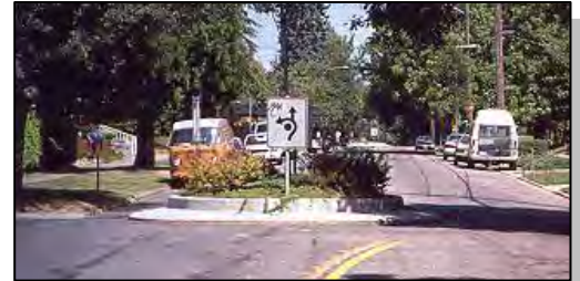
Example: Vertical inner curb and mountable apron.
