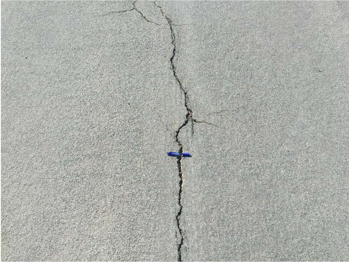
Photograph No. 2: Typical Taxiway J, G, D, and P distresses
