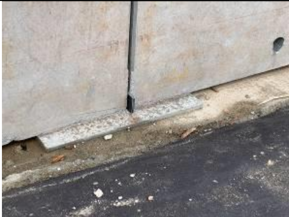
Setting pads for walls over footings
