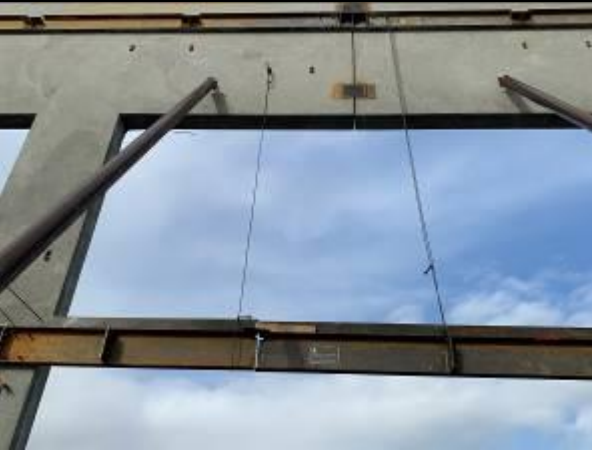
Temporary connection of floor ledger between wall panels
