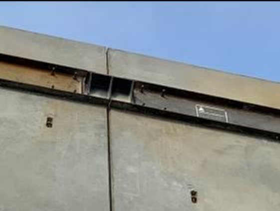
Roof truss beam seat welded onto wall panels
