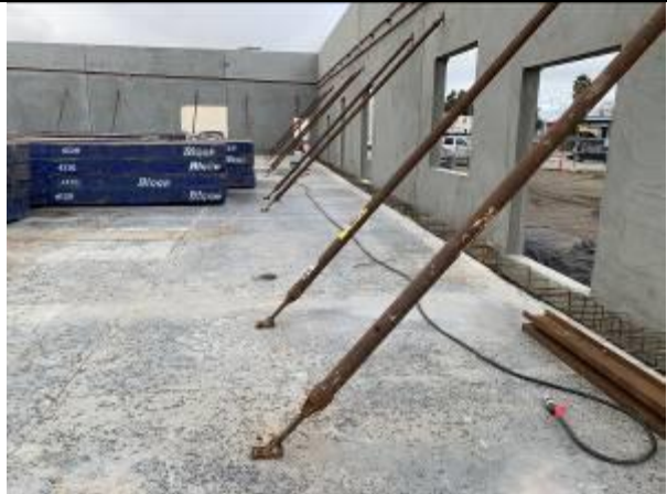
Temporary braces support wall panels
