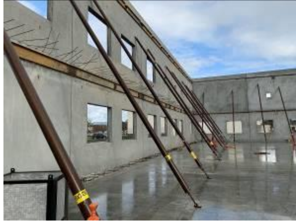
Two story walls temporarily braced
