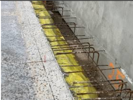
"Closure slab" area between walls and floor slab
