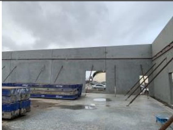
Steel ledgers installed for roof truss support
