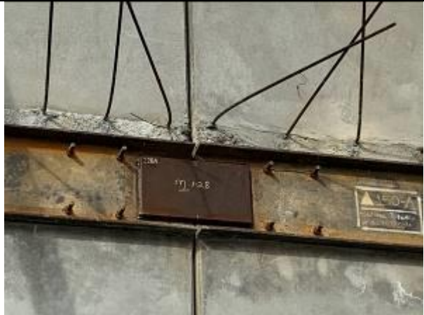
Final welded panel connection with steel plate
