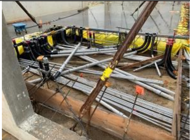
Electrical room conduit in place
