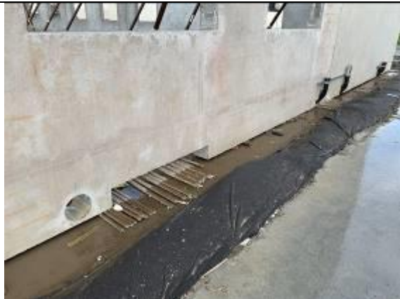
Low voltage service conduit installed to HQ
