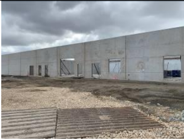
Support Building Walls tilted into place
