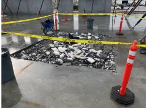
Removing slab concrete for elevator pit
