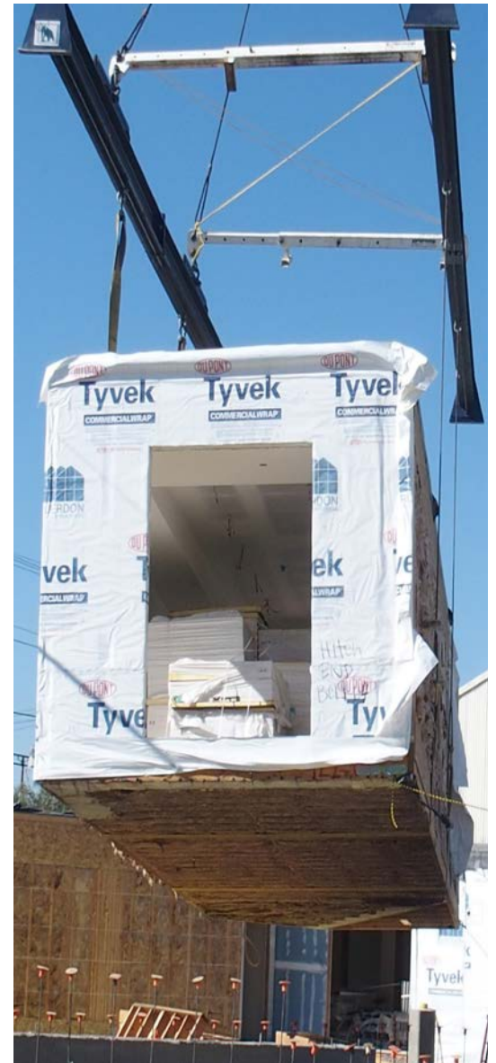
Hikari Apartments modular unit being dropped into place along the building's foundation.
