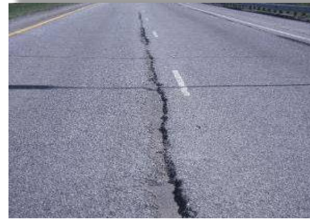
Transverse or Longitudinal Cracking
