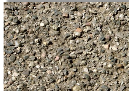
Weathering or Raveling
