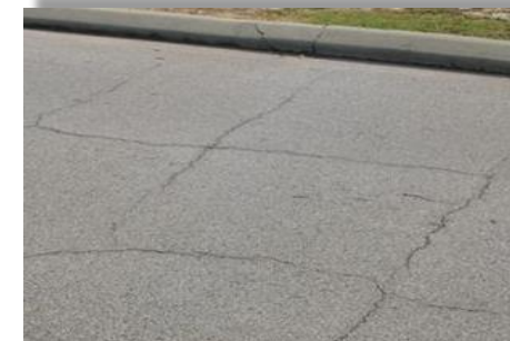
Block Cracking
