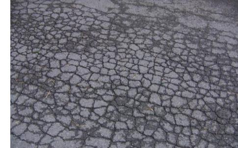
Alligator Cracking
